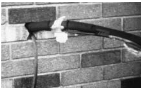
Common entry point for mice, rats, ground squirrels, birds and other small animals. Better attention should be paid to utility line entry points.
